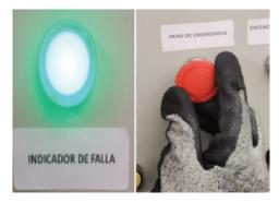
In case of failure, the indicator will illuminate.
