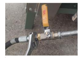
Connect the gas hose and stopcock at the inlet of the carburetor valve
