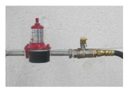
Connect to a gas outlet with high-pressure regulator.
