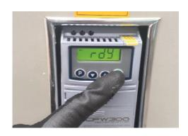
Press the ON button (green) of the speed drive to turn on the main motor.
