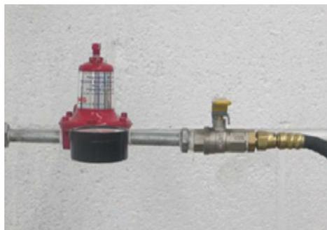
**6** Connect the high pressure regulator (2403) to the gas connection outlet.
