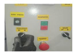
Activate temperature control switch OFF/ON. 3 OFF indicator will turn on (red light)
