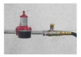
Connect to gas outlet with high pressure regulator.
