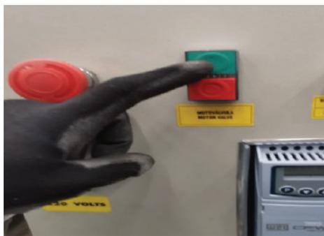
**12** Activate the ignition button of the motor valve.
