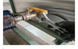
Ensure gas intake tightening to prevent leaks
