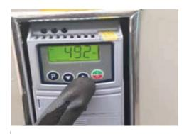
Modify the working speed of the metal bands by pressing the speed drive buttons.
